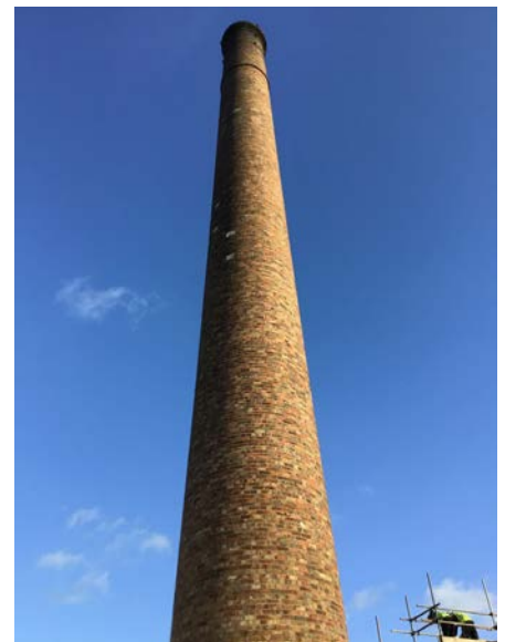
Glengall Road Chimney
