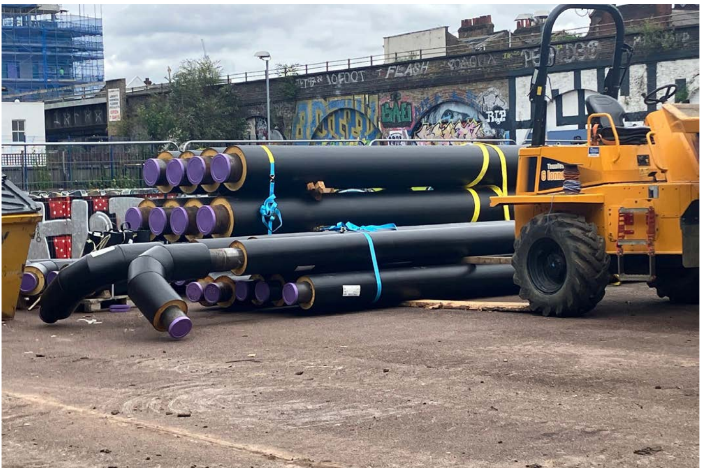
District Heat Network pipes on site at Brimington Park prior to installation
