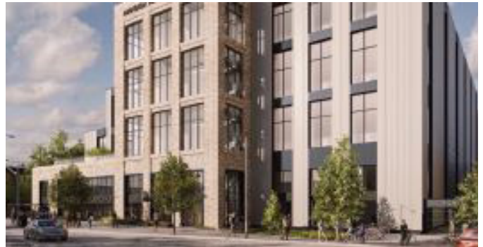
25 Mandela Way - Stacked logistics hub
